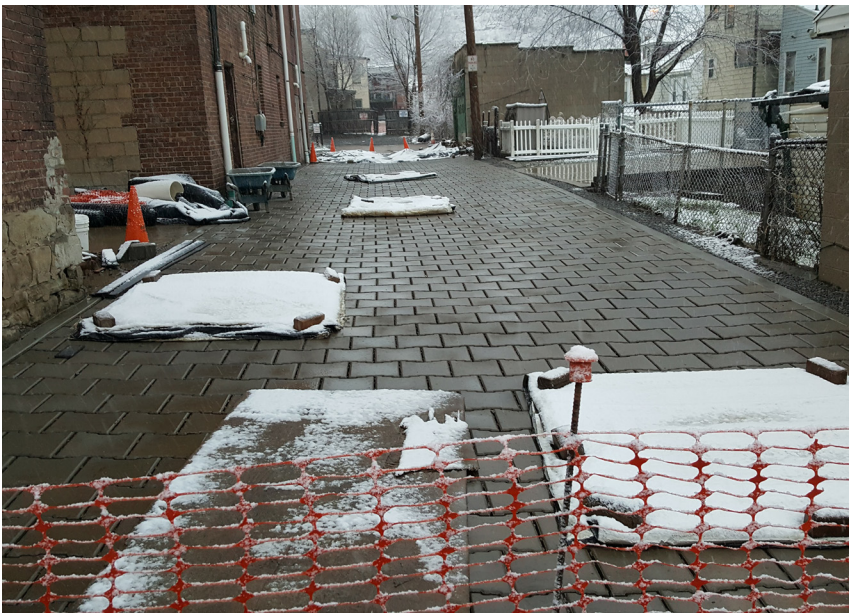
Permeable Pavers as part of a Green Stormwater Master Plan. Source: The Philadelphia Water Department
