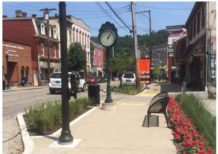
Trench drains and rain gardens add to the streetscape in Etna, Pennsylvania. Source: Etna Borough
