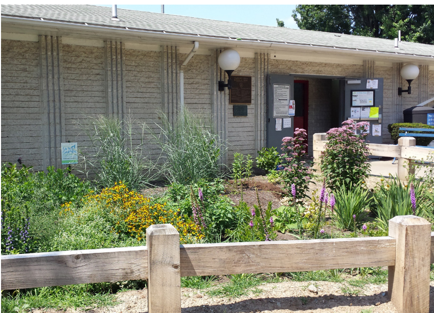
Playground rain garden. Source: The Philadelphia Water Department
